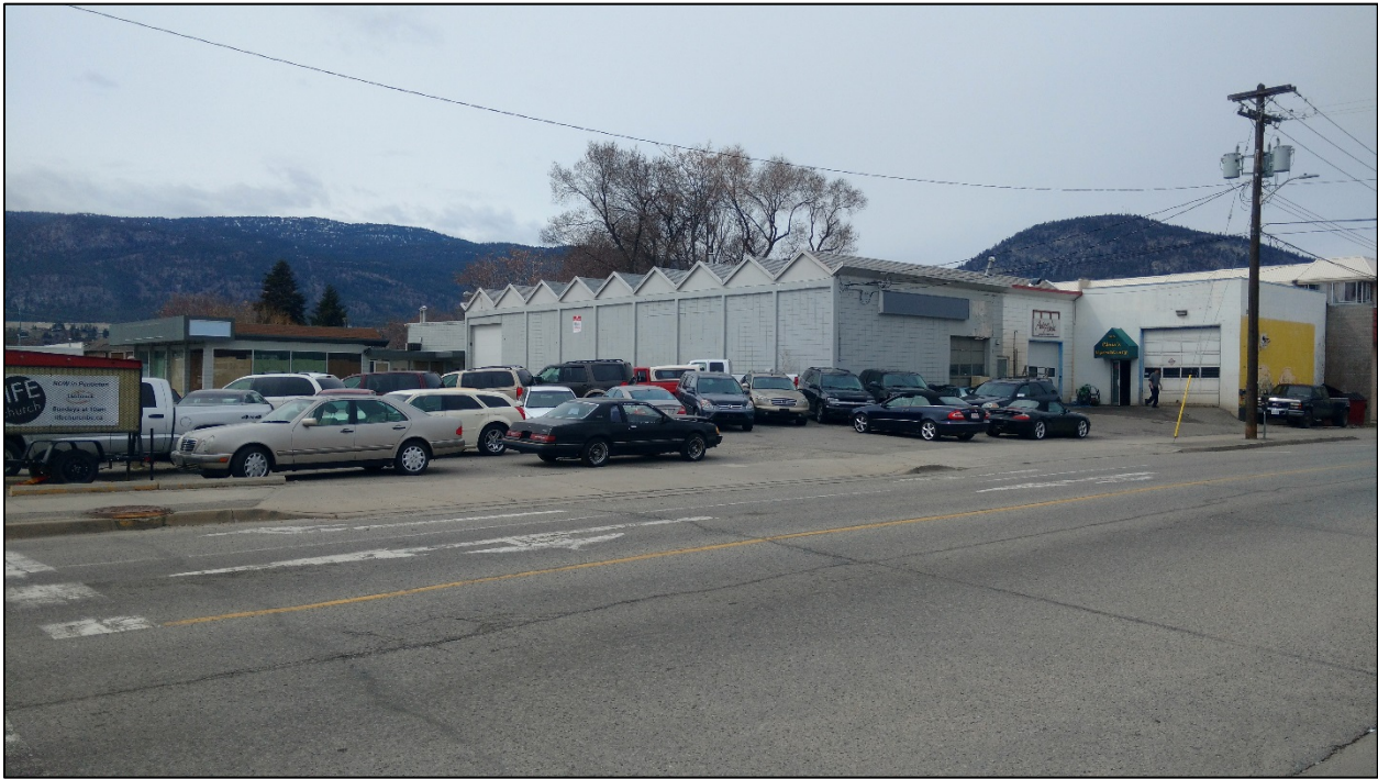
Figure 5: East View (from Winnipeg Street)
