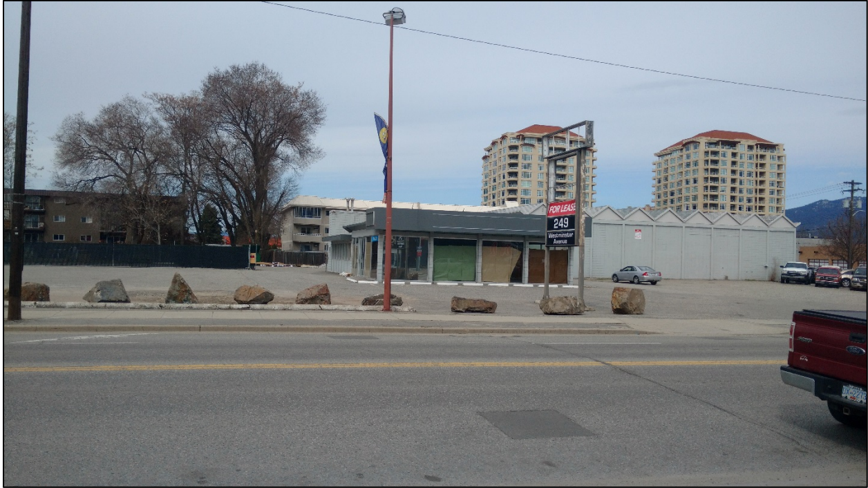
Figure 7: South View of Subject Property
